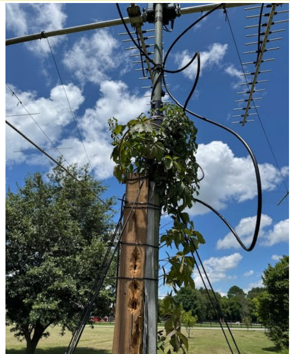
The pileated woodpecker (left) has done extensive damage to Steve's antenna supports (above, closeup below)
