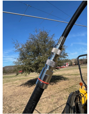
Steve installed a new Heliac connector
