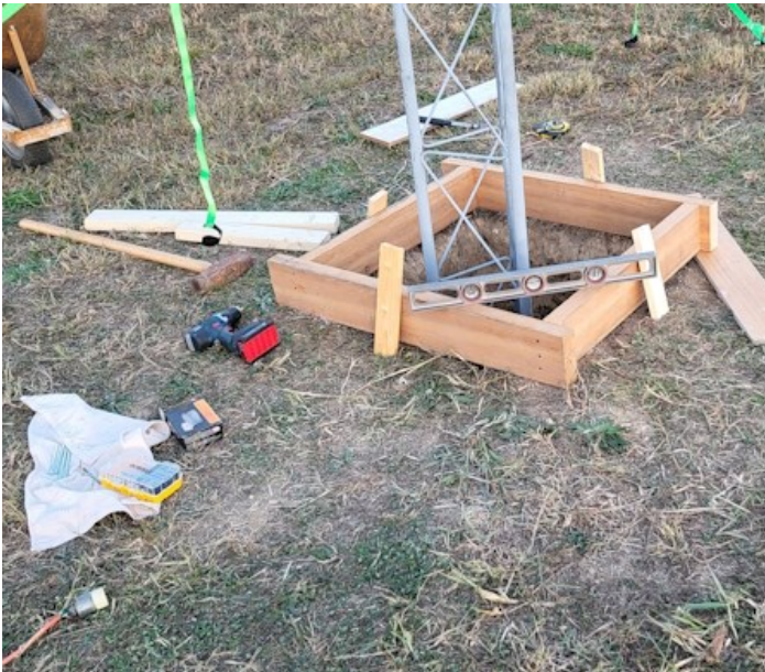
Above: The sloped form for the concrete base.
