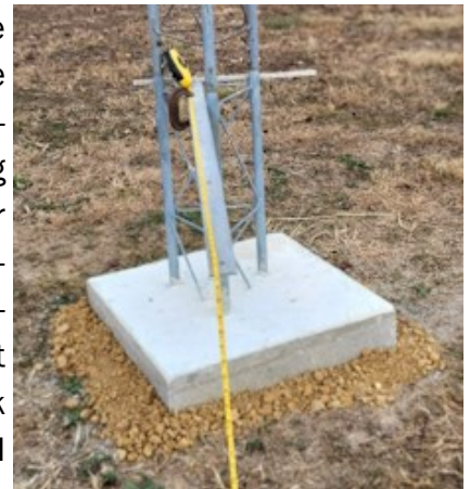
Rohn tower specs allow only 5 degrees off-axis so a 4' metal T-square was used to precisely set the anchor locations.
