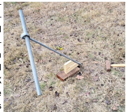
Rohn tower specs allow only 5 degrees off-axis so a 4' metal T-square was used to precisely set the anchor locations.
