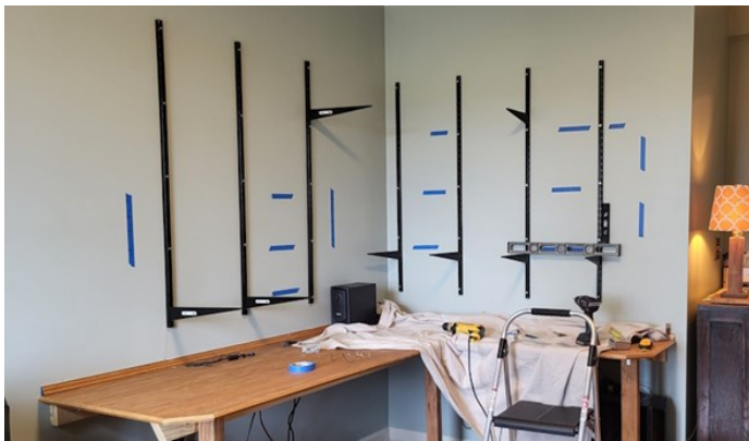
Shelving was added and anchored into studs.
