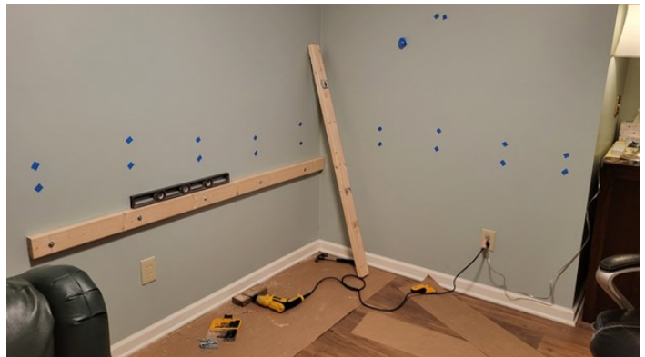
Studs were used to anchor the desk to the wall.
