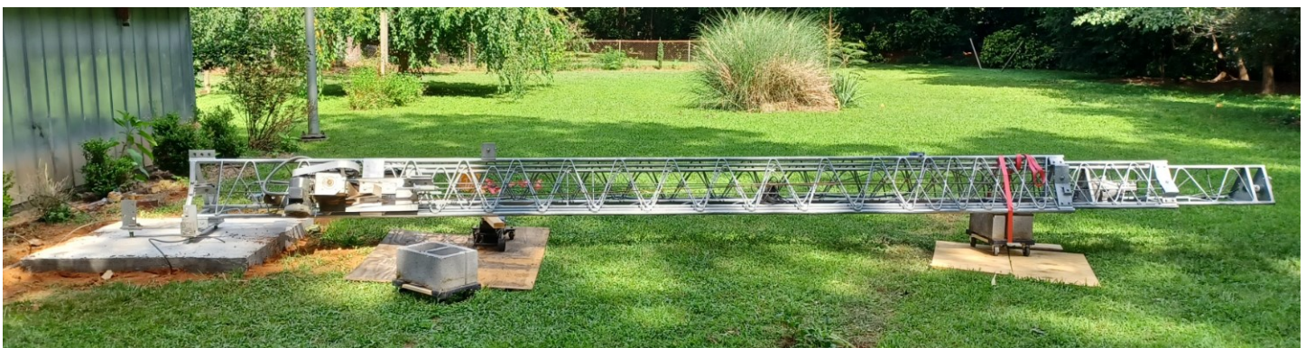
The tower was moved into position by placing furniture dollies underneath and making a plywood path.
