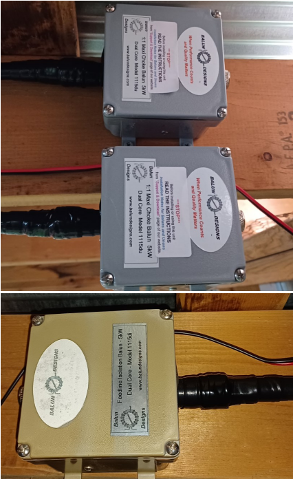
Above: Baluns are installed on each coax run.
