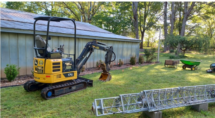
The rented excavator made digging a lot easier.
