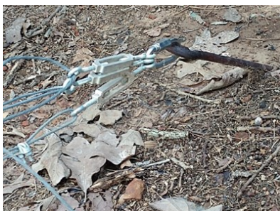
Guy anchor and turnbuckles
