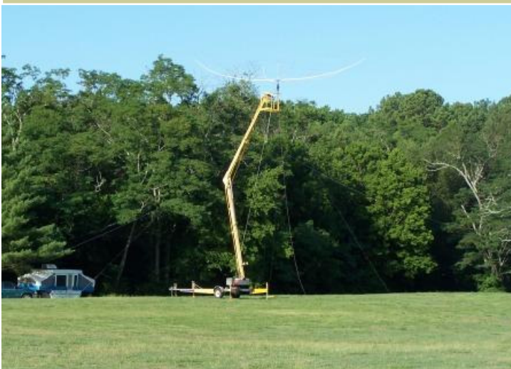
Taking the cue from Decatur FD last year, Barry, W4WB, uses a lift to support the 40m SSB hexbeam and dipole.
